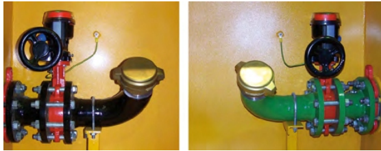
Fig. 2.2 Refueling ports of diesel fuel (left) and petrol incl. vapour recovery (right)
